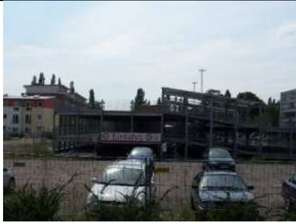
Figure 3-22 Stellwerk 60 Car Park
