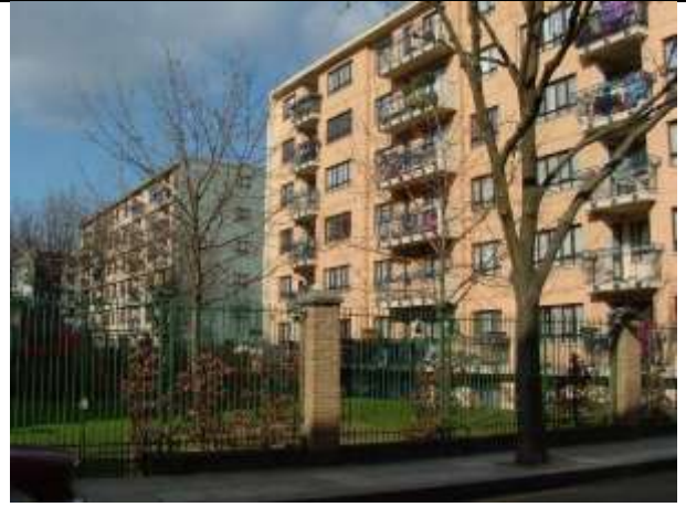
Figure 6-6 Council flats, Kings Cross Ward
