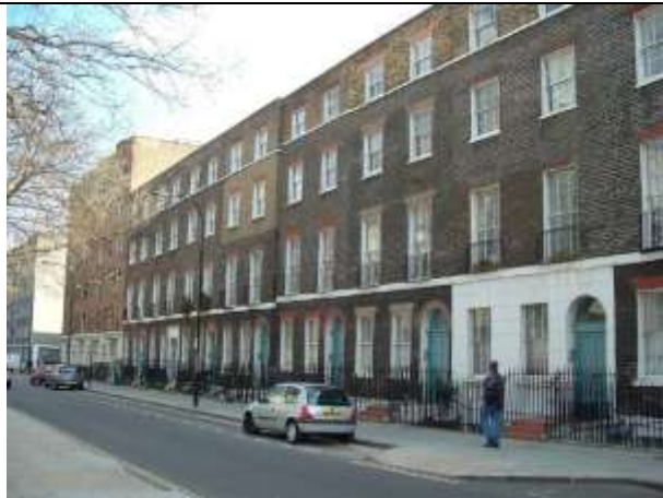
Figure 6-7 Terraces converted to flats, Bernard St., Bloomsbury Ward
