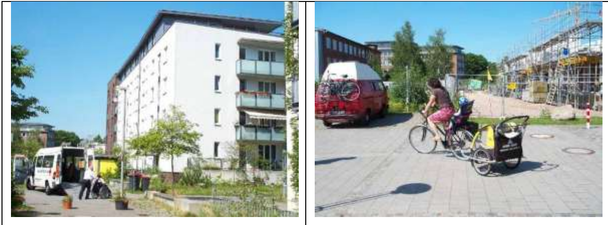
Figure 3-16 Saarlandstrasse phase 1 and phase 2 under construction
